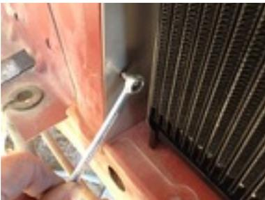
When it is slid all the way in, attach the front plate to the front wall of the cavity with two of the #10 hexhead sheet metal screws.
